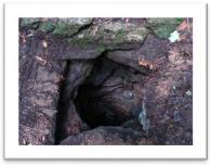
ily drew drinking water from a 27-foot-deep well to the left of the house. To build a well, settlers dug a large coneshaped hole. Once enough water was found, a circular stone wall was built in the hole and backfilled with packed dirt.
